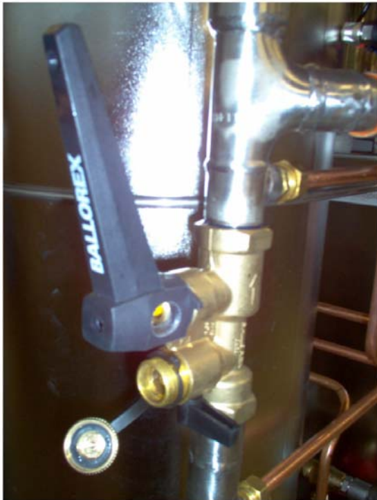
Ball valve on adjustment valve #27
