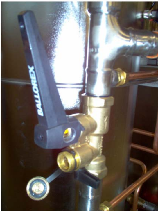
Ball valve on adjustment valve #27
